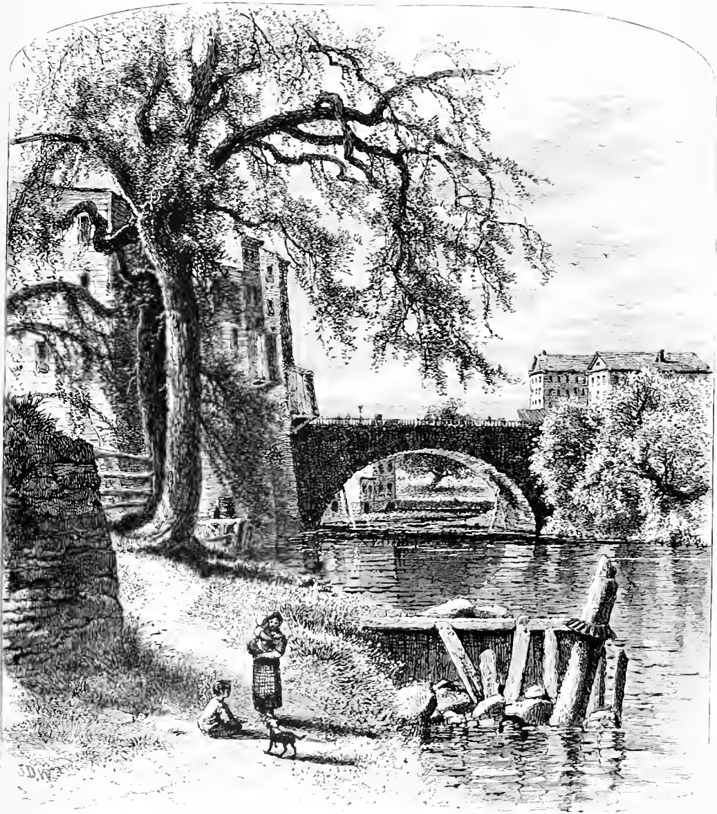
Main-Street Bridge, Hartford
